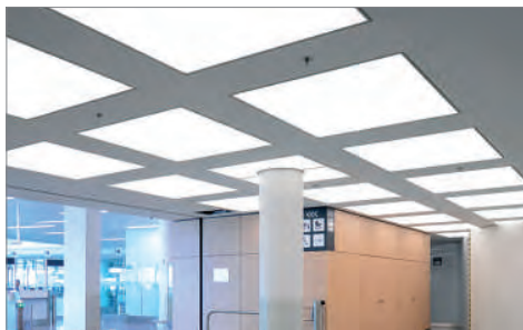
Arch. : Chapman Taylor architects - Plafond lumineux - Luminous ceiling - Leuchtende Decke
