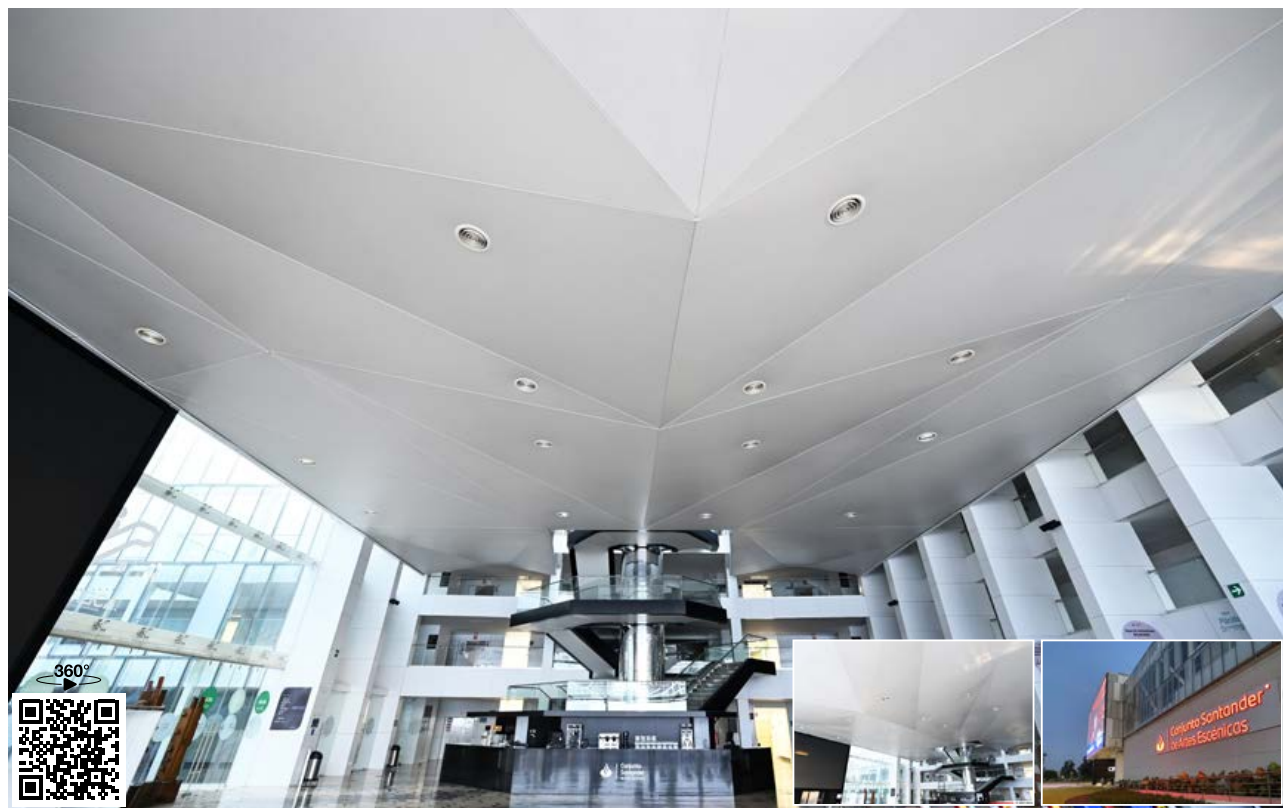
Barrisol® Formes 3D | Barrisol® 3D Shapes Arch. : Cristian Ezcurdia - Jaume Soler (ARUP)
